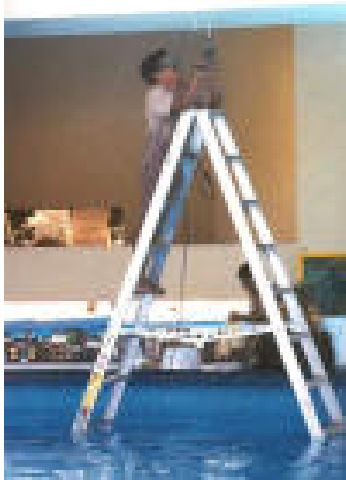
Ladder in water with electrical drill
