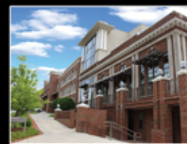
Montgomery County Commission Offices Renov. Montgomery, Alabama
