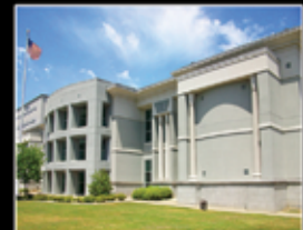
Etowah County Judicial Building Gadsden, Alabama
