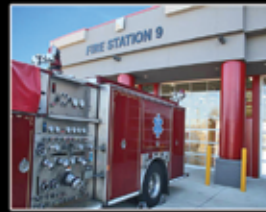
Montgomery Police & Fire South Precinct Montgomery, Alabama
