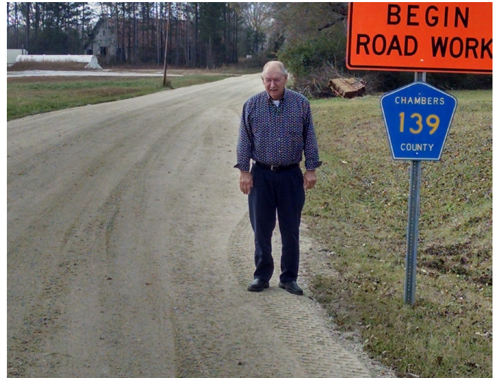
AFTER | Gravel Surface
