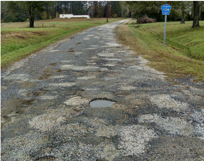
BEFORE | Paved Surface
