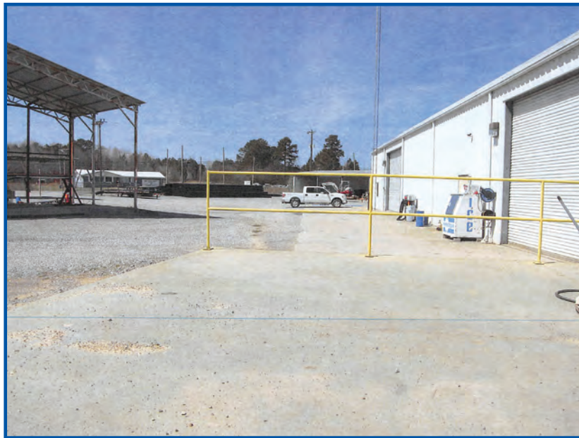
The water department uses this concrete platform for pressure-washing equipment, and one side of the platform is above grade. Employees recognized the uneven work surface as a safety risk, and as a result they installed this new yellow guardrail
