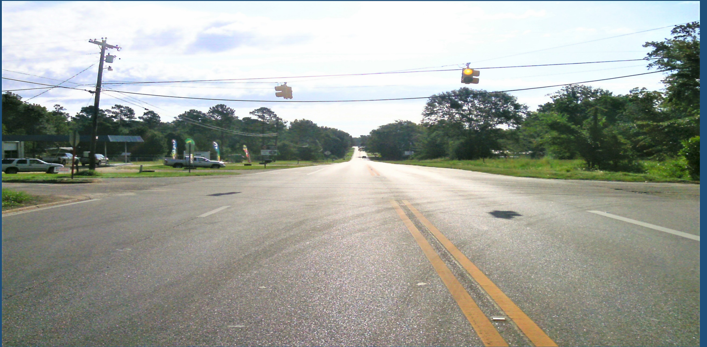
State Route 52 - County Road 69 Intersection - Looking East
