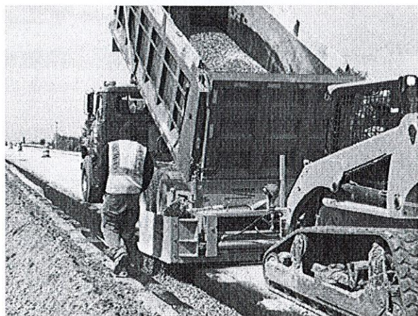
Trench backfilling with the FH Model.
