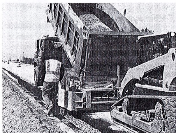
Trench backfilling with the FH Model.
