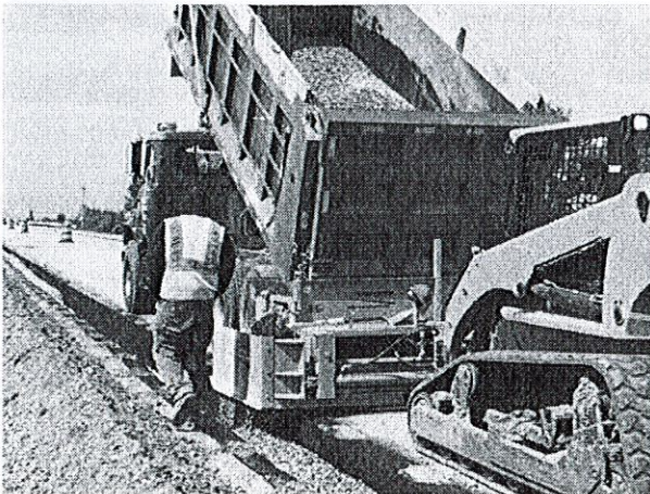
Trench backfilling with the FH Model.
