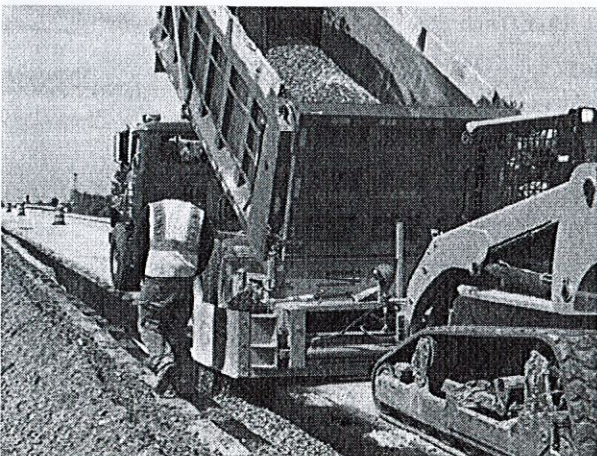
Trench backfilling with the FH Model.
