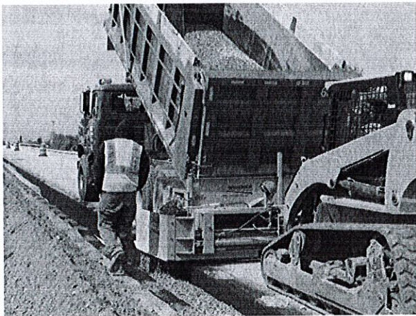
Trench backfilling with the FH Model.
