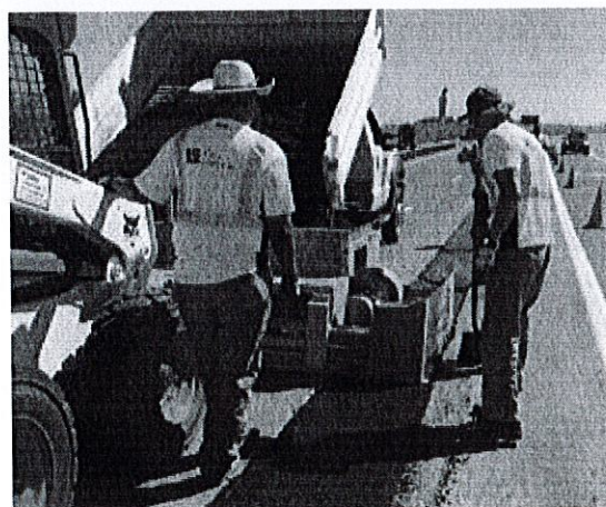
"Mill and fill" has never been easier.
