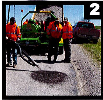
Inject Emulsion Aggregate Mixture
