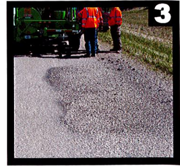
Cover With Dry Aggregate
